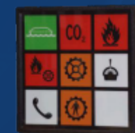
LSD 210.80.0.1 indication panel
